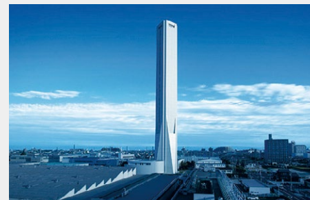
SOLAÉ elevator testing tower
