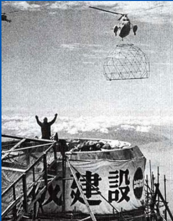
The radar dome reaching the summit in 1964 amid turbulence – even veteran pilots feared for their lives. (Photo: Mitsubishi Electric)
