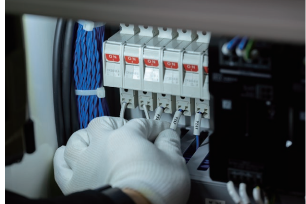
For switchgear and breakers with spring clamp terminals, the connection is completed by inserting the wire.
