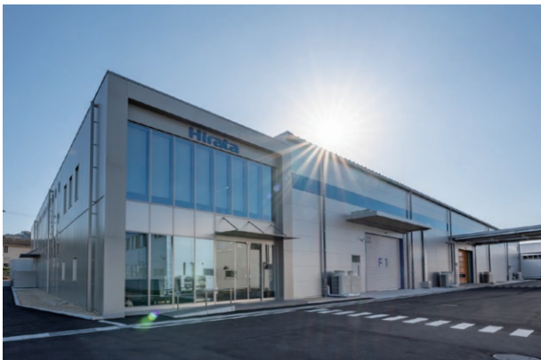
Hirata Corporation's Kansai Plant where Mitsubishi Electric's electrical switchgear fitted with spring clamp electrical terminals are bringing multiple benefits.
