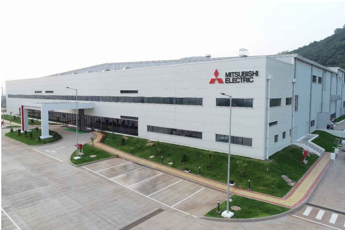
Mitsubishi Electric's new manufacturing plant for factory automation systems in Maharashtra, India
