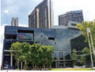
Thailand FA Center MITSUBISHI ELECTRIC FACTORY AUTOMATION (THAILAND) CO.,LTD
