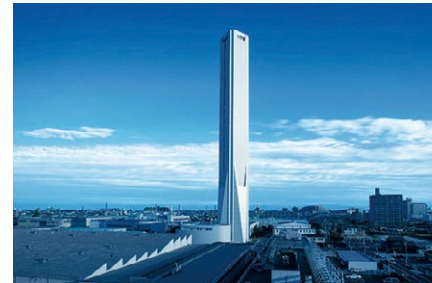
SOLAÉ elevator testing tower
