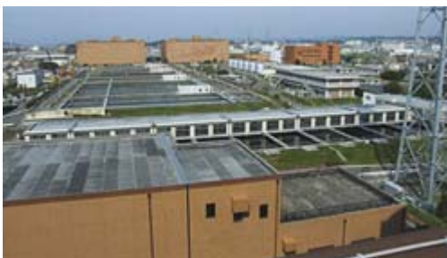
Murano Water Purification Plant
