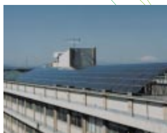
Photovoltaic Power Generation System
