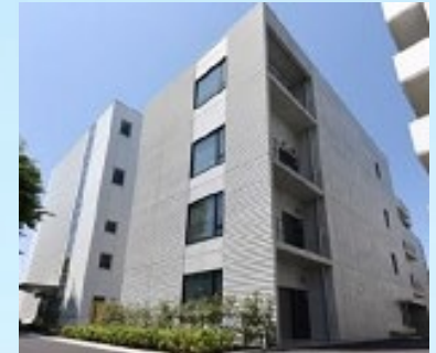
Modernization Training Building "Ren" Mitsubishi Electric Building-Techno Service
