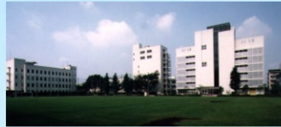
Educational Center Mitsubishi Electric Building-Techno Service
